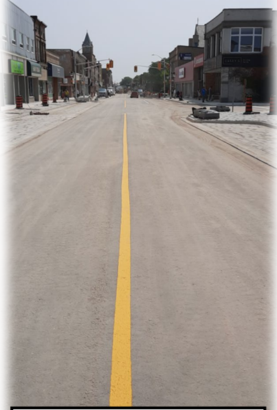
Talbot Street Stage 1 looking East towards Hiawatha
